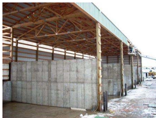
Bunker with Roof (Latah Co., ID.)
