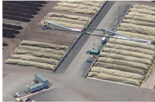
Membrane covered system (Everett, WA.)
