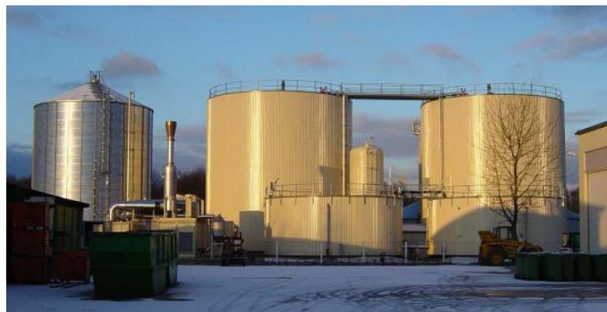
Wet anaerobic system (Germany)
