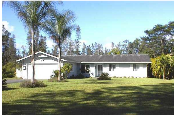
Residential development in the Hawaiian Shores subdivision.
